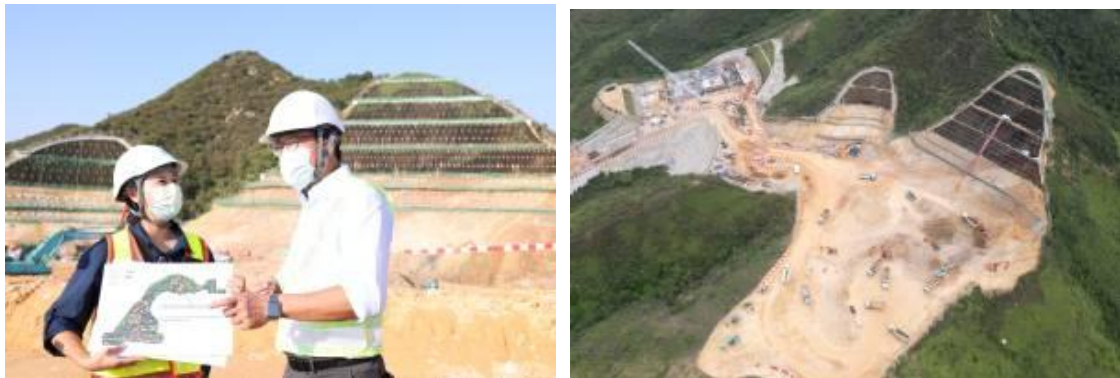
Cuttings and site formation at Tai Shek Mo (source: DevB)
